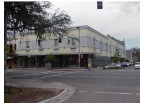
Existing Court Services Building
