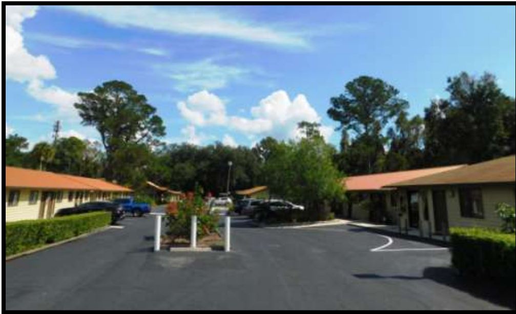
View of buildings - from front entry/access
