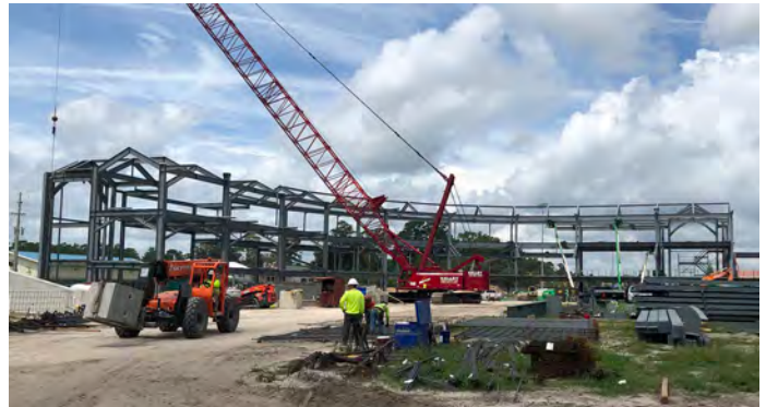
Florida Ballpark - Under Construction
