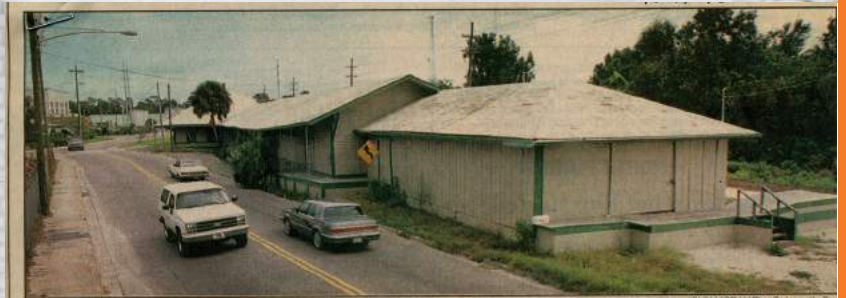
The old railroad depot on Depot Avenue could become a museum, the core of a project that would incorporate a stormwater retention lake and wetland to the south. The entire area would serve as a park.
