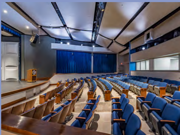
Santa Fe College Building E Auditorium Renovation
