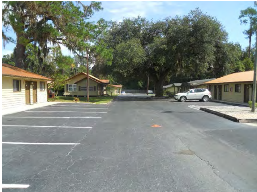
View of the subject driveway and parking area looking east towards the rear of the property.
