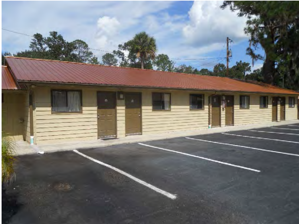
View of a typical subject building.
