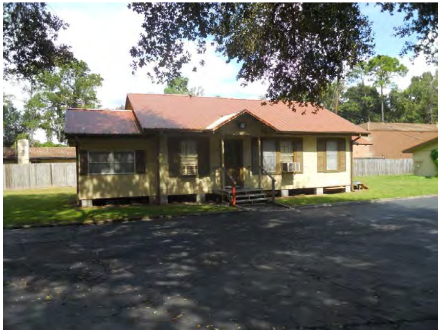
View of the exterior of the single-family house.
