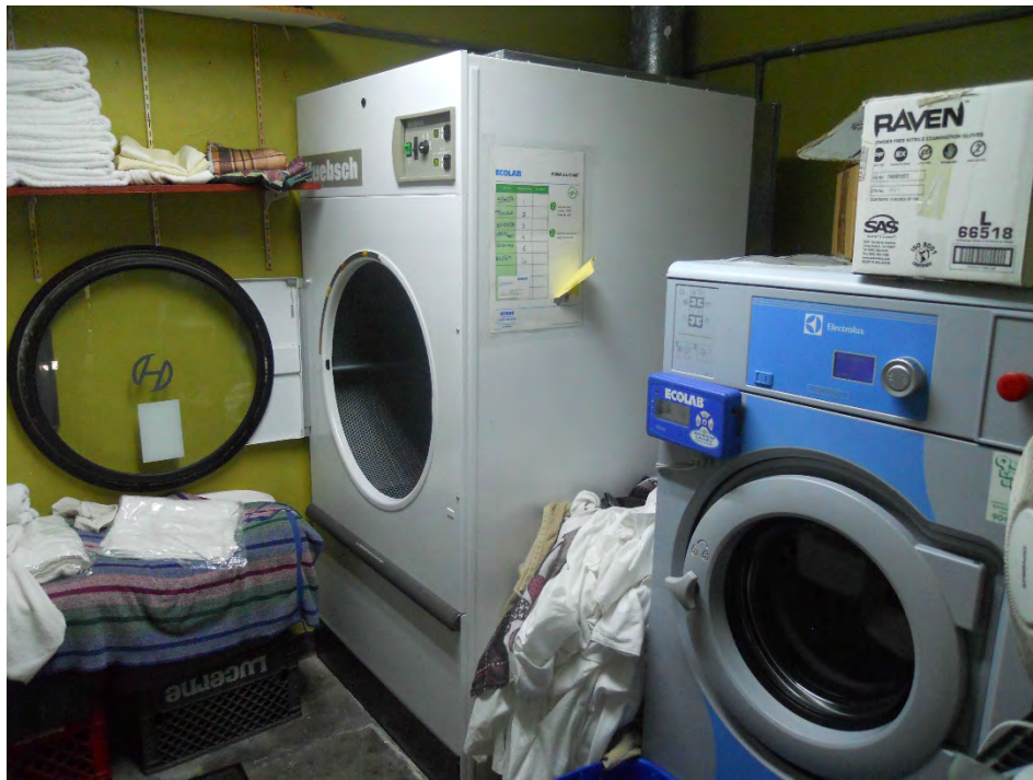
View of the laundry room within managers unit.
