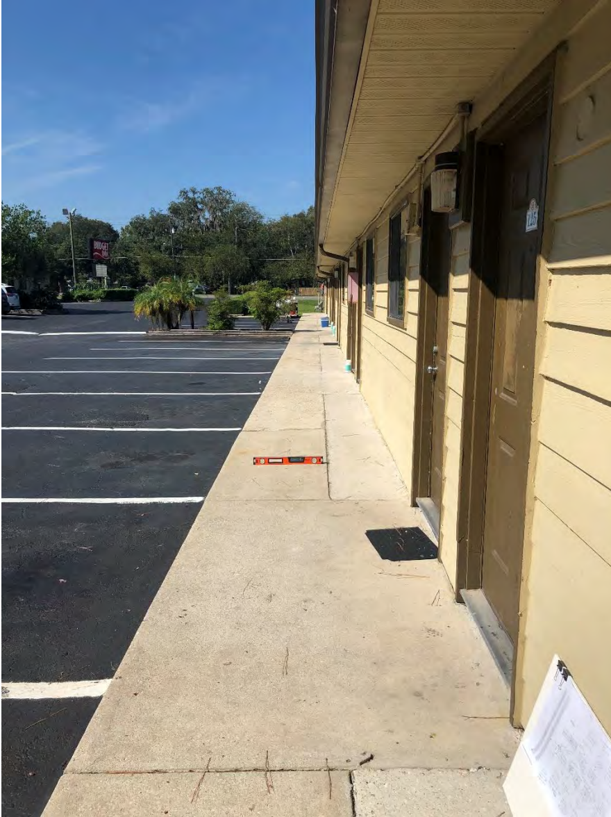
Figure 18 - South Side of Buildings 7 and 8
