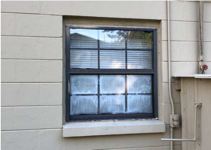
Figure 9 - West Window Building 4
