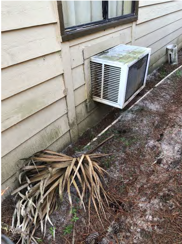
Figure 16 - North Side of Building 7
