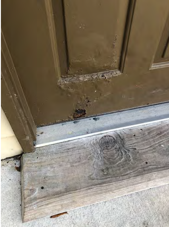
Figure 7 - Door at Unit 109
