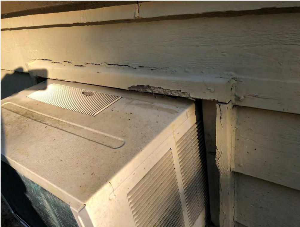
Figure 4 - Trim at AC Unit Building 1
