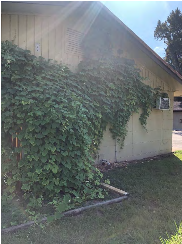
Figure 14 - West Wall Building 5
