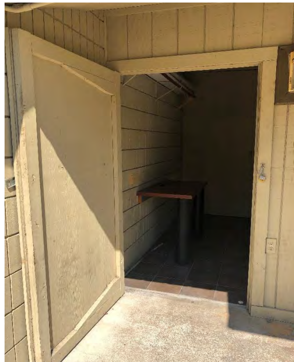
Figure 17 - Storage Area between Buildings 7 and 8
