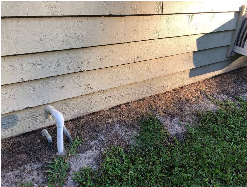
Figure 3 - Siding on Building 1
