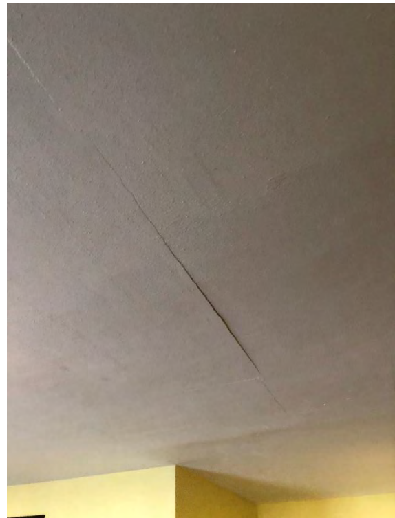
Figure 8 - Ceiling at Unit 112
