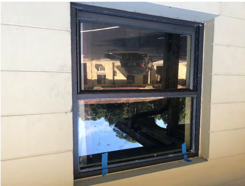
Figure 10 - Window Repair Building 4
