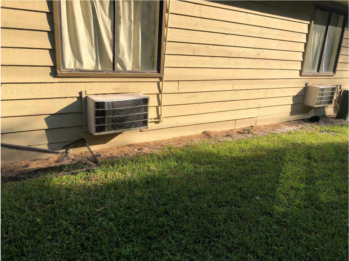
Figure 6 - Grade at Building 2
