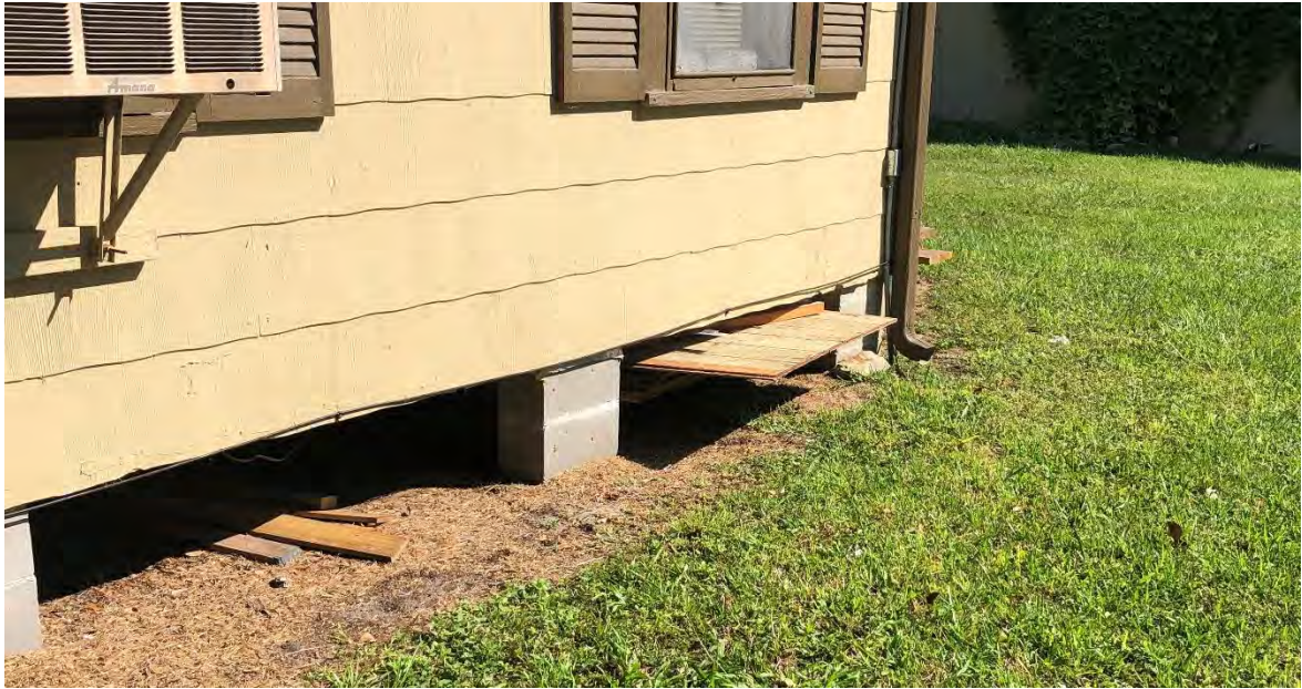
Figure 15 - Crawlspace at Building 6
