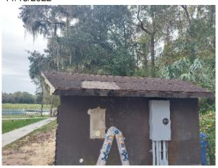
Dry area as needed. Embed existing granules as needed. Prime affected area. Apply new modified bitumen cap sheet in cold-process adhesive to affected area per manufacturer's recommendations.
