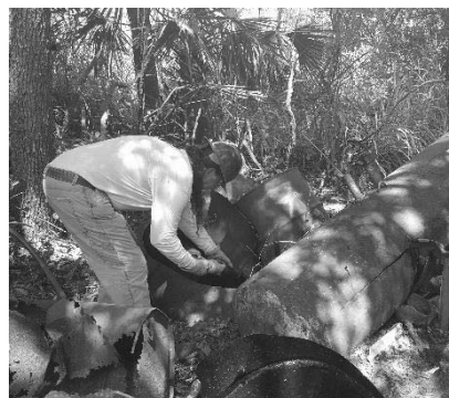
Geosyntec provided oversight as environmental construction contractors removed product from the abandoned tanks/drums, cut them into pieces and disposed of them properly.
