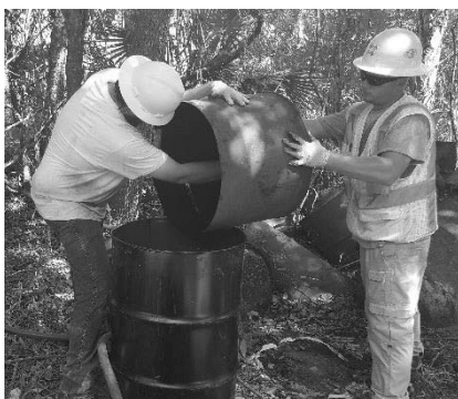
Geosyntec provided oversight as environmental construction contractors removed product from the abandoned tanks/drums, cut them into pieces and disposed of them properly.
