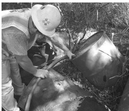
Geosyntec provided oversight as environmental construction contractors removed product from the abandoned tanks/drums, cut them into pieces and disposed of them properly.
