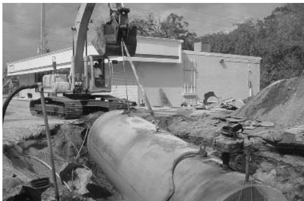
UST Tank Removal and Excavation at Cumberland Farms #0955
