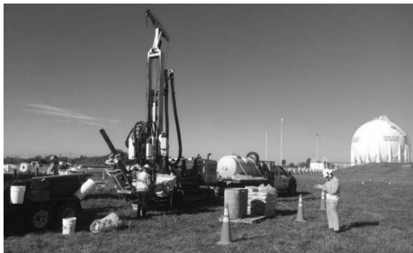
Air Sparge and Monitoring Well Installations at LC-39B
