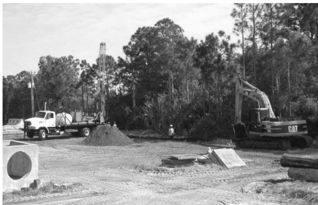
Remediation wells being installed at the South Gifford Road Landfill Site, in support of the selected remediation strategy.
