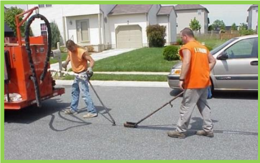
Crack Sealing
