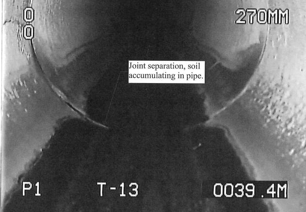
© 270MM | End of pipe joint cracked.
