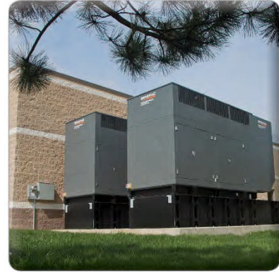
Figure 12. Backup Power Generators
