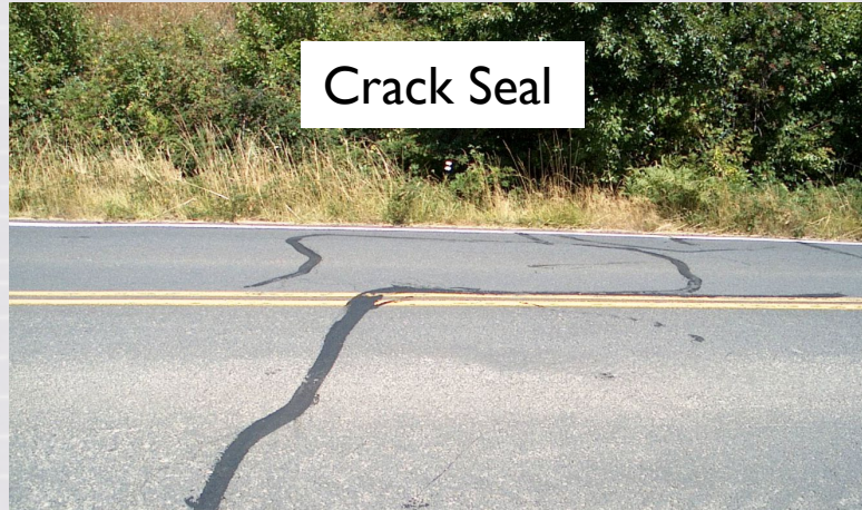
Poor Practice Crack Seal
