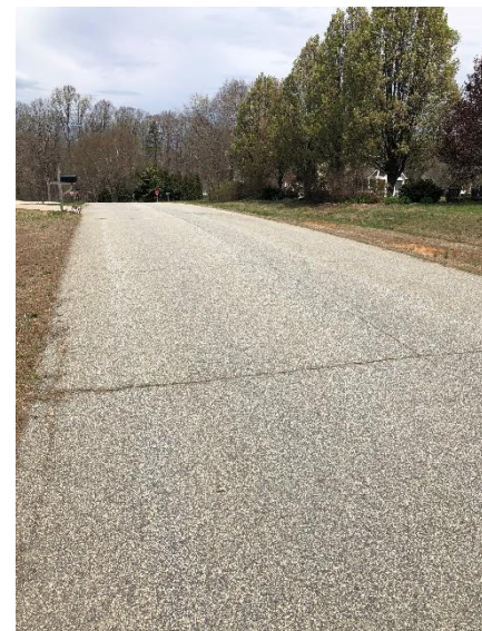
Transverse Cracking.
