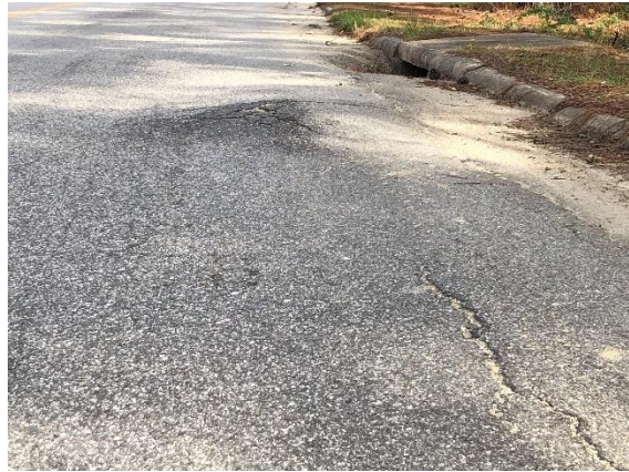
Medium Severity Roughness
