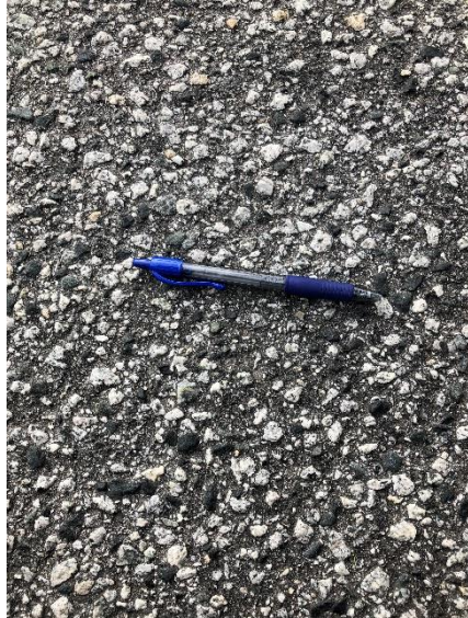
Medium Severity Raveling
