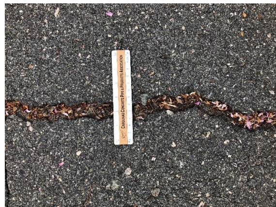
High Severity Transverse Cracking.
