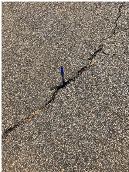
Medium Severity Transverse Cracking.
