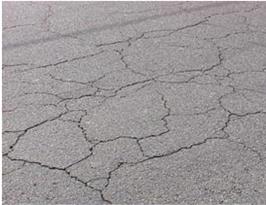
Medium Severity Block Cracking
