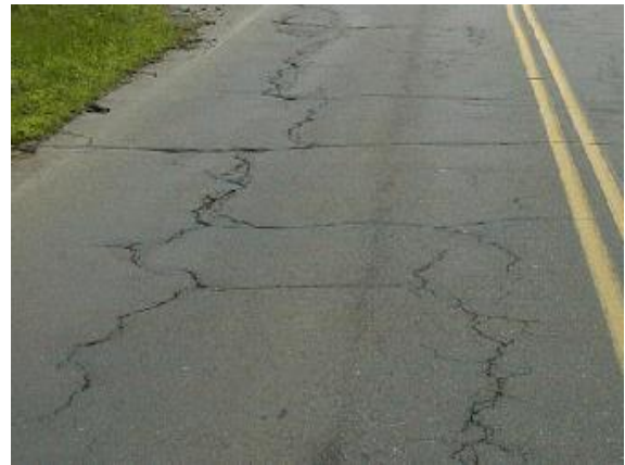
High Severity Block Cracking
