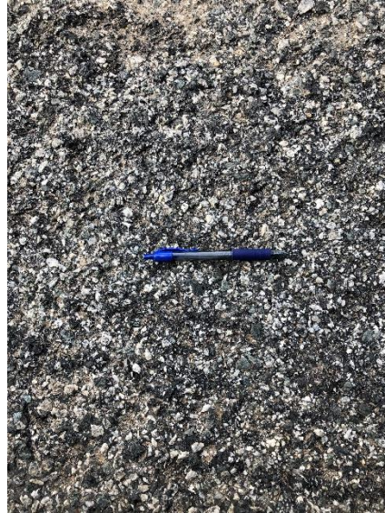
High Severity Raveling
