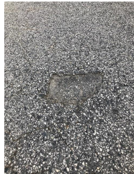
Medium Severity Pothole
