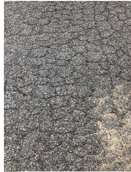
High Severity Fatigue Cracking.
