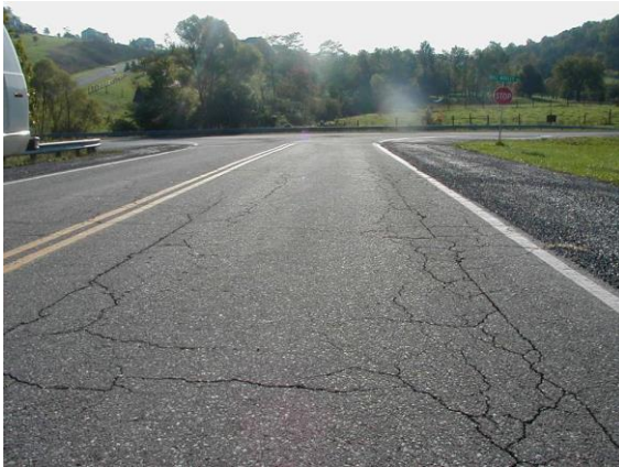
Medium Severity Fatigue Cracking.
