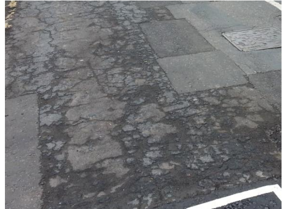
High Severity Patch
