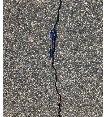
Low Severity Transverse Cracking.
